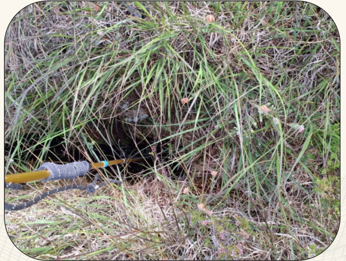
Bell profile drain void hiding a drain c.80cm deep and fast flowing
